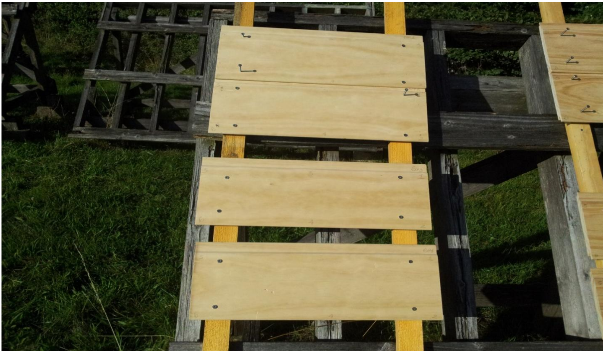
Photograph 1. Arrangement of cladding on the rigs with boards fixed to the battens at 400mm centres.
