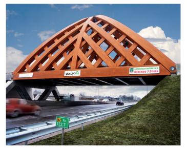
Figure 7: A large scale application of  $\mathsf{Accoya}(\ensuremath{\mathbb{B}}$  wood – Sneek bridge, the Netherlands
