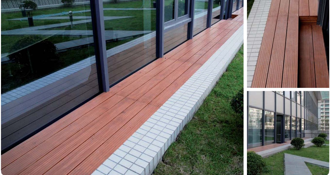
Decking for the roof garden of Baidu Search Engine's R&D Centre, Shanghai
