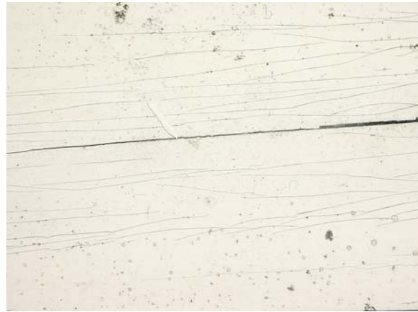
Wood cracks, cracks in the coating and degradation of the coating layer by blue stain fungi of acetylated (with residual acetic acid) Scots pine finished with an opaque white alkyd coating after 9½ years outdoor exposure (sample 36102).
