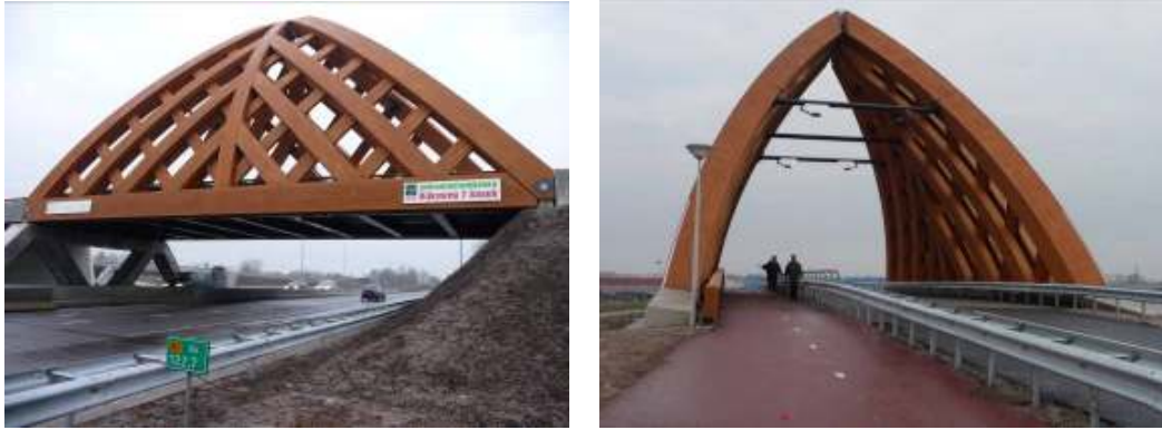
Figure 12: A large scale application of Accoya® wood – Sneek bridge, the Netherlands
